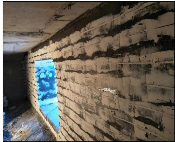
Fig 13. Laminate Fixing and Application of Putty
