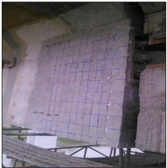
(b) Marking on New Concrete for Grooving
