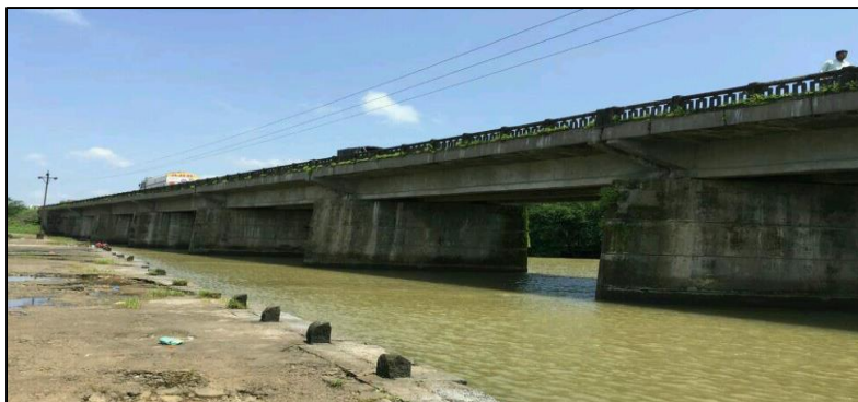
Fig 7. Dharna River Bridge at Ghoti, Nasik
