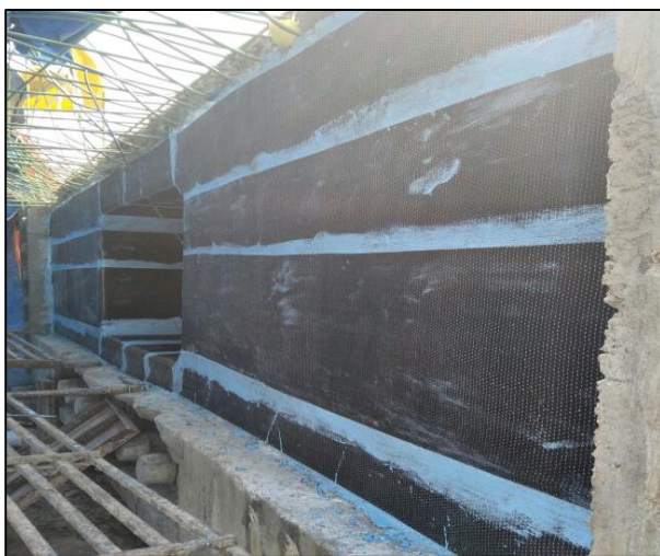
Fig 14. Application of FRP to Increase Strength
