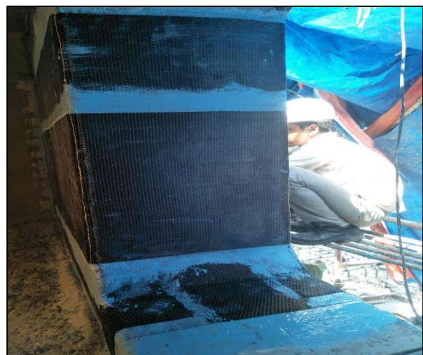
Fig 14. Application of FRP to Increase Strength
