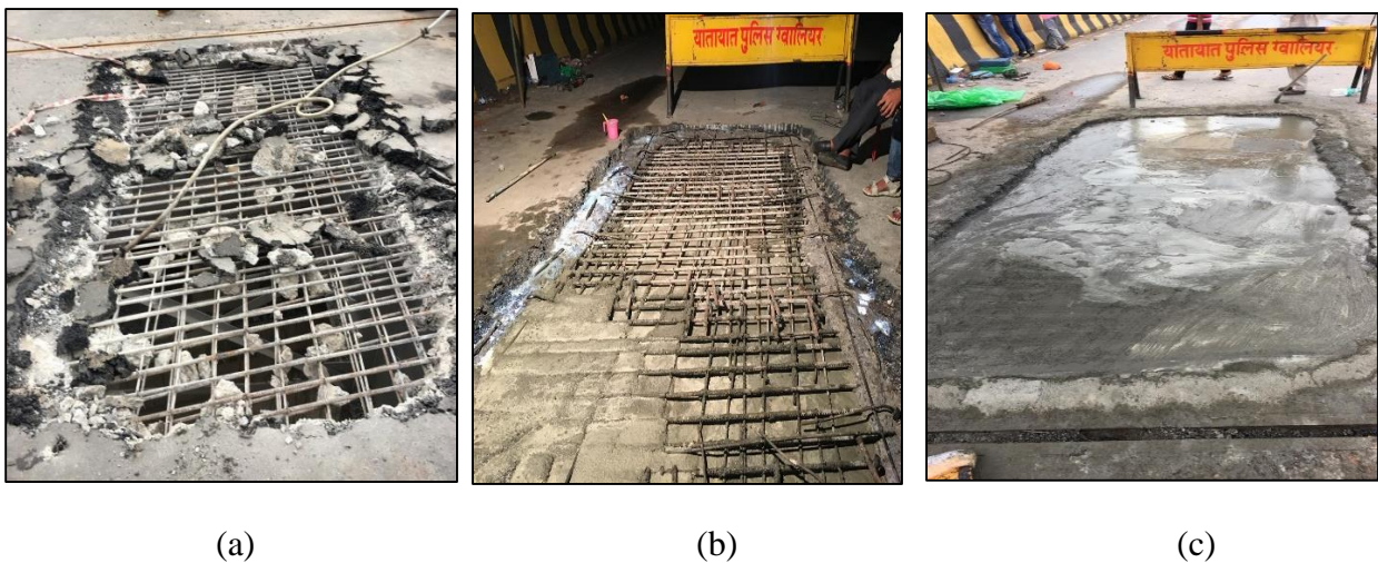
Fig 17. (a) Removal of Damaged Concrete (b) Micro -concreting with Bonding Agent (c) Curing of Concrete
