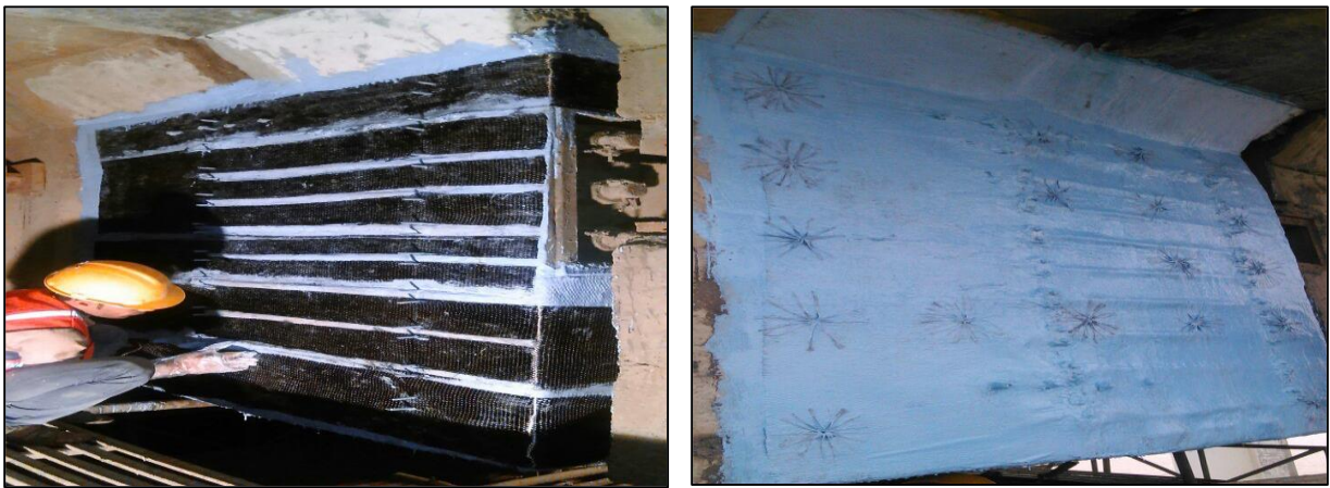
Fig 6. FRP Strengthening of Bridge's Hinge Connection Part
