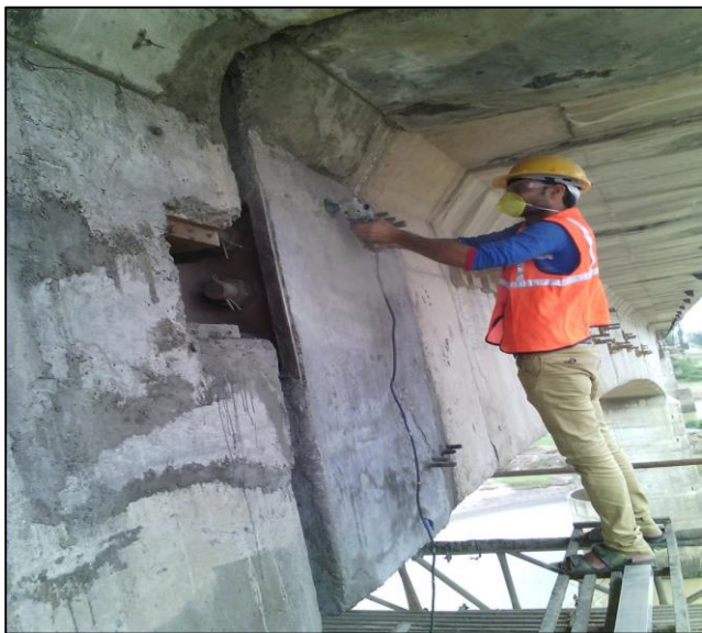
(a) Grinding of New Concrete Surface Preparation
