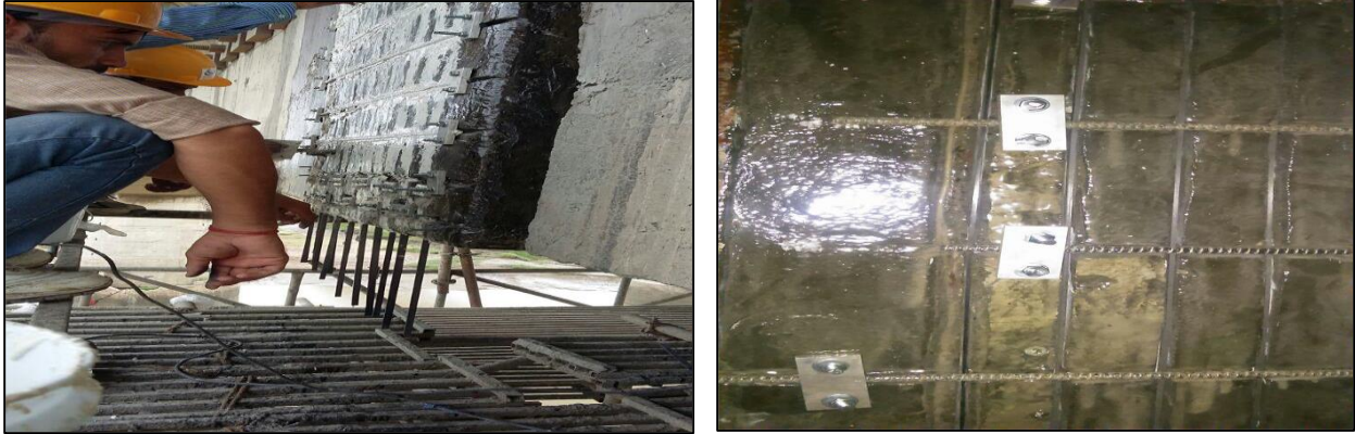
Fig 5. Fixing Additional Reinforcement on Concrete surface
