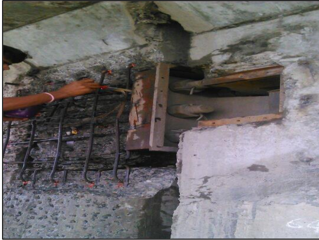
(a) Anti-rust application on exposed Reinforcement
