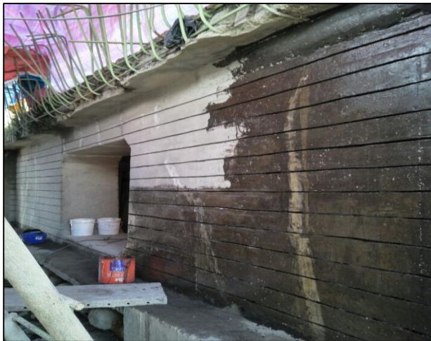
Fig 12. Grooving and Primer Application
